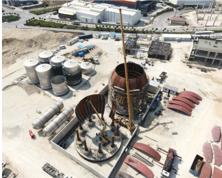
Tank and steel erection
