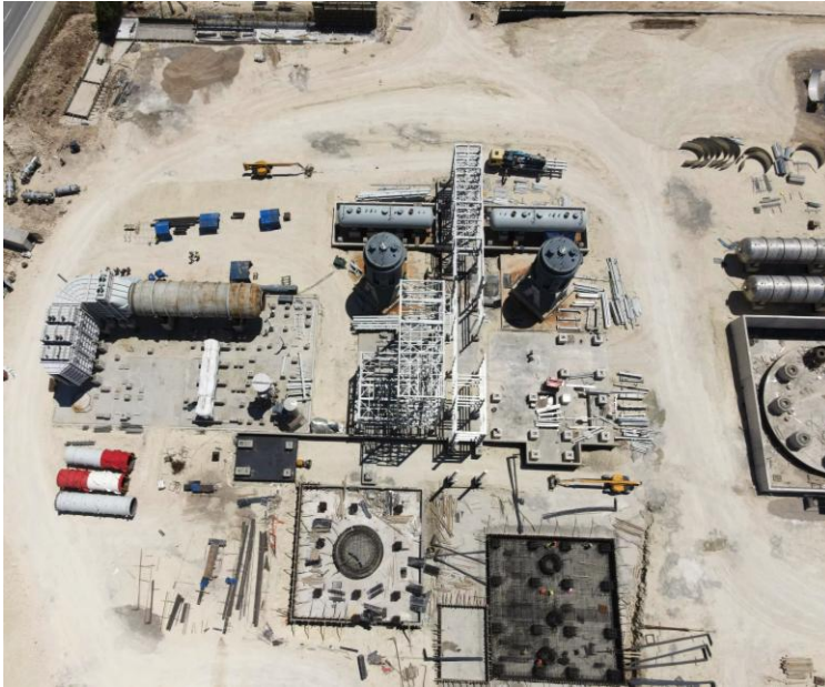
Early civil works
