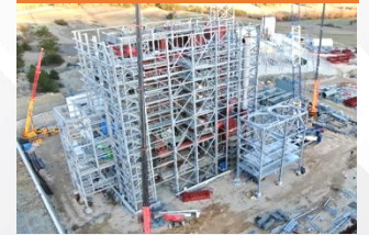
CONSTRUCTION & CIVIL WORKS
