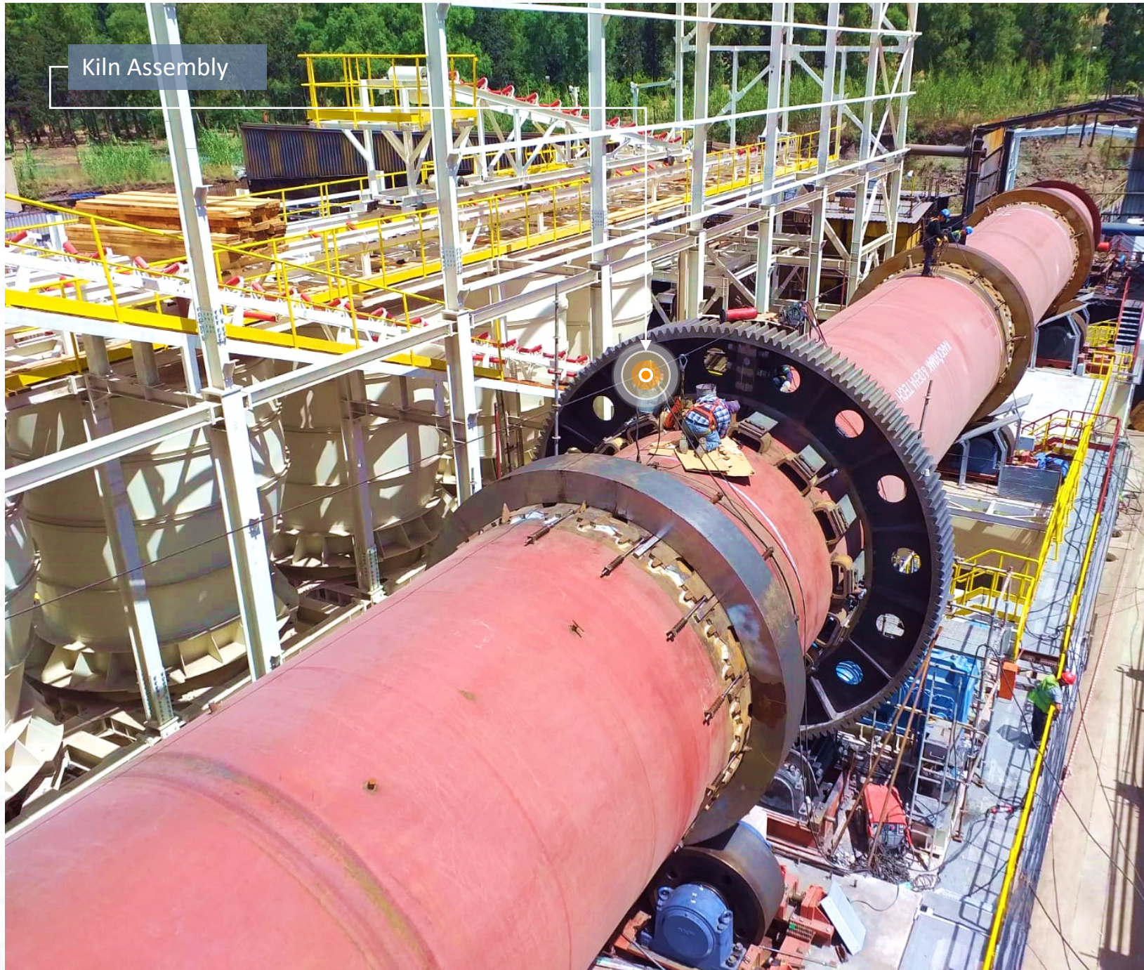
Kiln Roller Assembly
