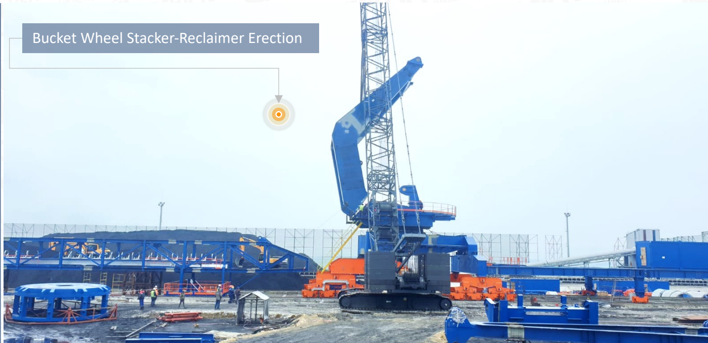
Bucket wheel Stacker-Reclaimer Erection
