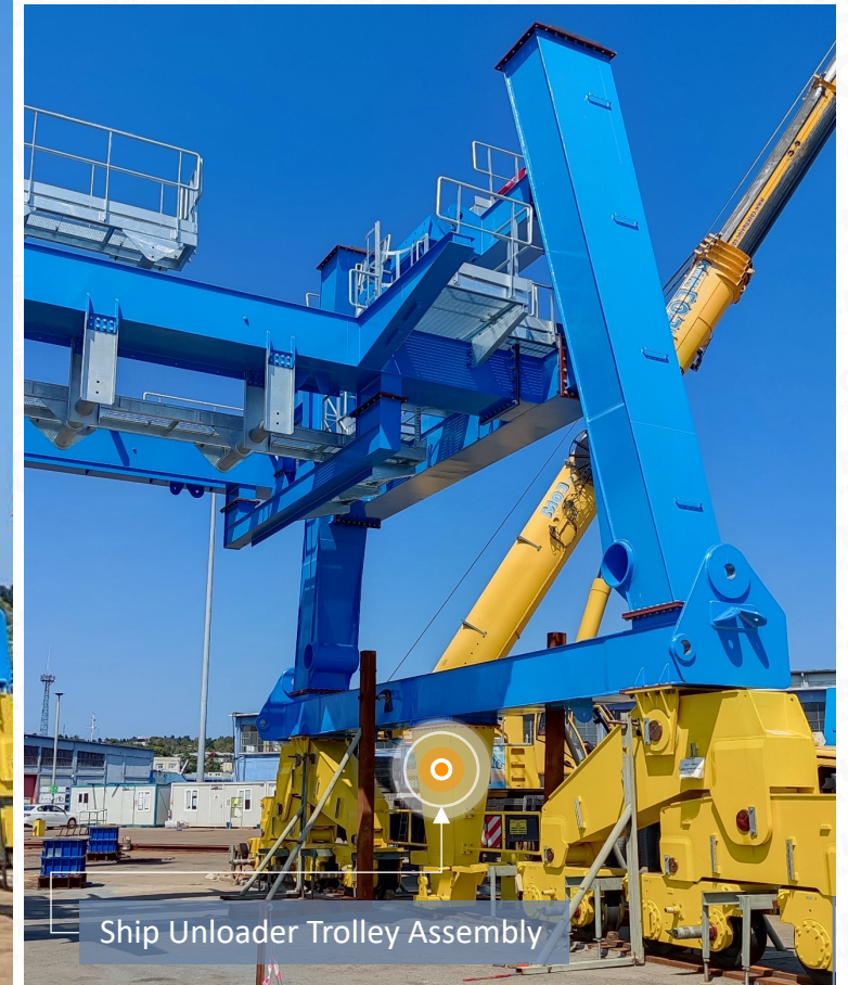
Ship Unloader Trolley Assembly
