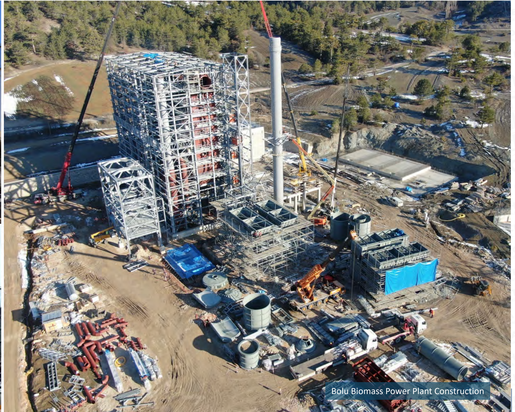
Ash Silo Bolu Biomass Power Plant
