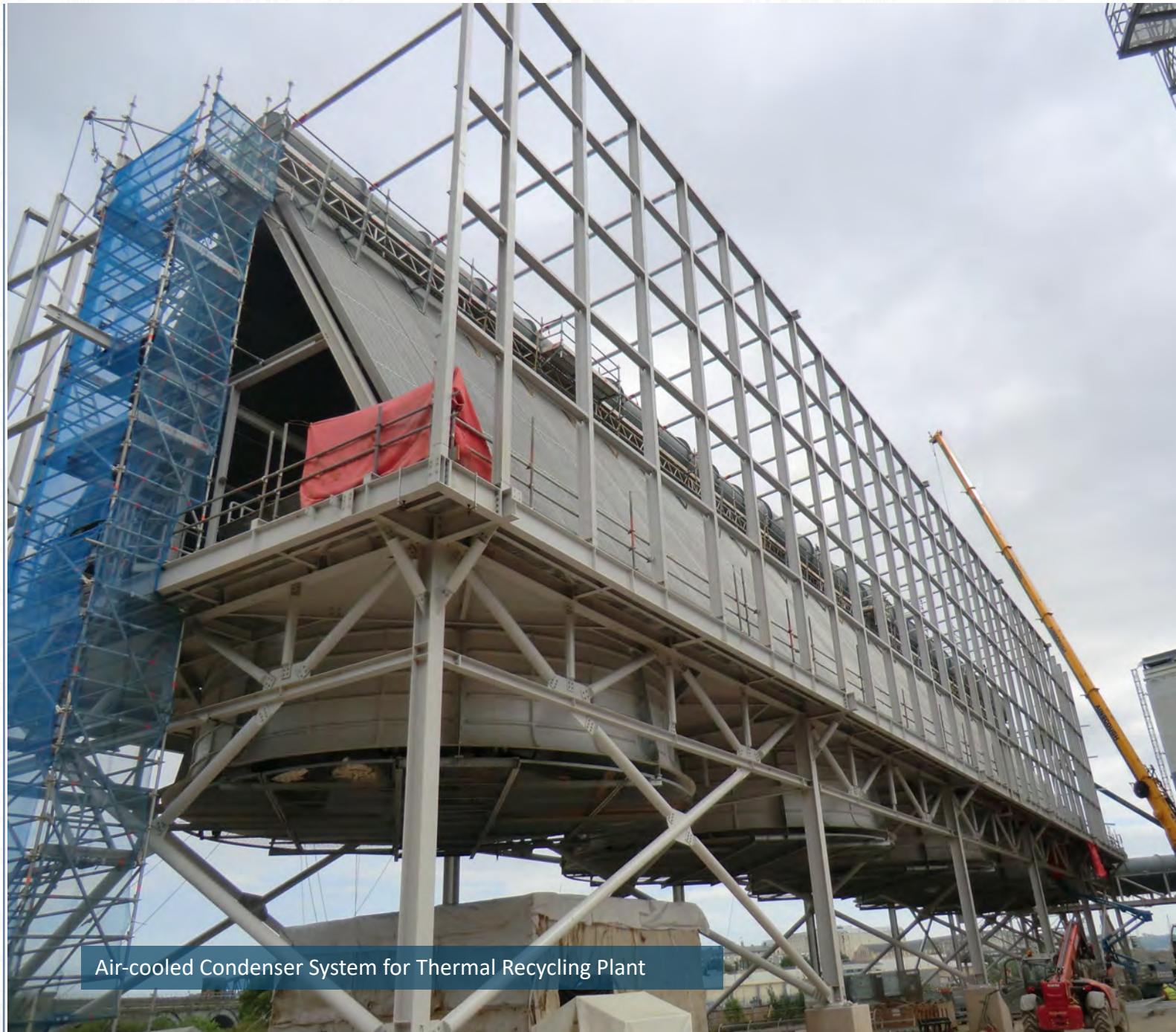
Prefabrication and Erection Cladding
