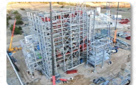
CONSTRUCTION & CIVIL WORKS
