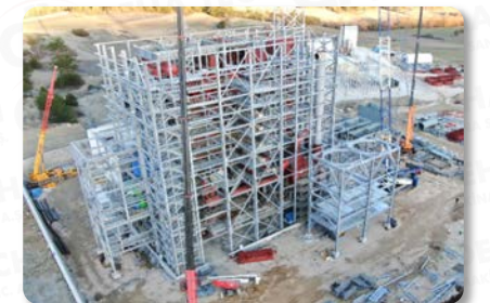
CONSTRUCTION & CIVIL WORKS
