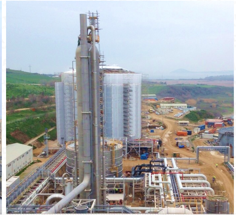
Bagfas Calcium Ammanium Urea Plant
