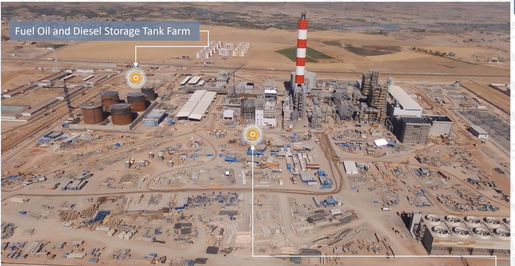
Limestone Storage Silo
